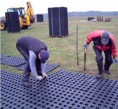
Sections arranged on the ground
