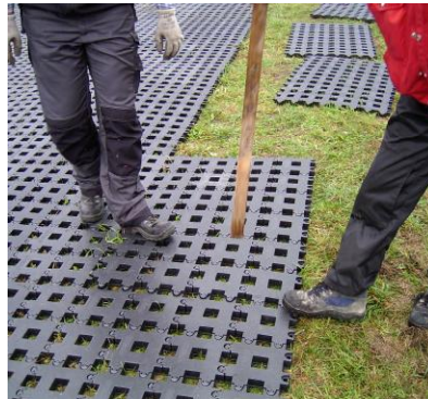
PERFO sections clipped together using foot pressure on
