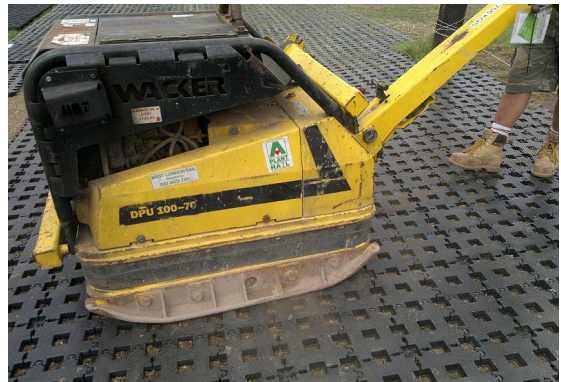
Heavy duty wacker plates or rammers can be used for initial compaction into the surface
