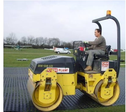
After about 3 rows are laid out, they should be rolled in leaving the last row unrolled.
